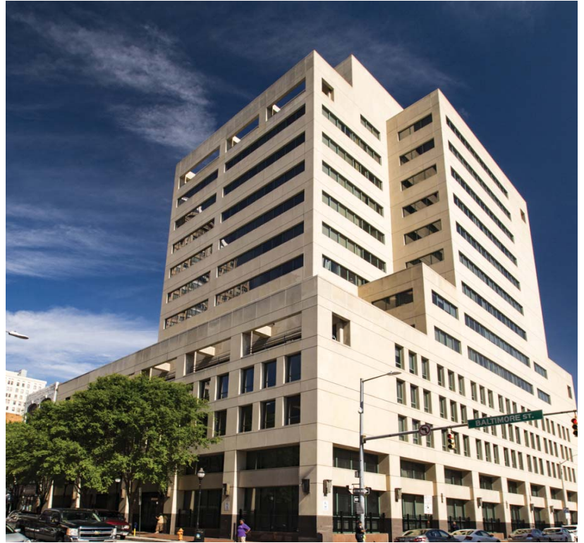
AFTER —The Benton Building cleaned, caulked, repaired, and sealed.
