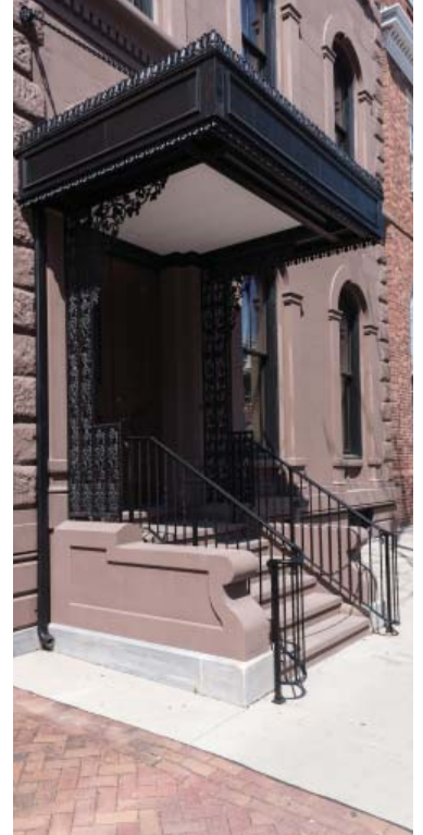
AFTER —The Market Street elevation included the replacement of 138 pieces of brownstone in 38 different profiles, shapes, and sizes.
