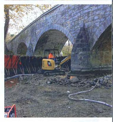
The initial design allowed for water seepage through the sediment, requiring the addition of seven water pumps. The solution included two large pumps for substantial standing water, along with up to five small pumps to remove puddled water. (The pumps continued to prove beneficial later in the project, being reversed-out to provide high pressure washing in prep for repointing, and to aid in cleaning.)
