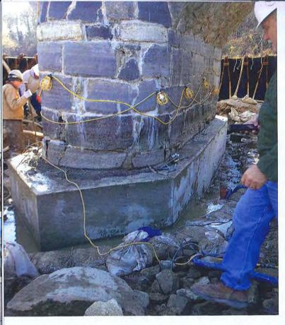
the piers. Once pumped dry, footing extents were wrapped in epoxy- coated rebar followed by forms. Witmer's crew poured new concrete footings for both piers – 8 cubic yards of concrete for each.
