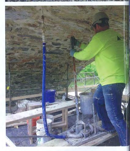
support. New slab was poured to encase the new and existing tie rods. With new footings, flowable fill stabilizing every crevasse, and the added tie rods, the piers' long-term structural integrity was assured.
